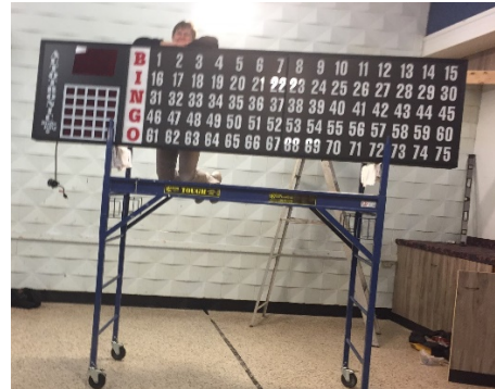
Heather assisting with installation
